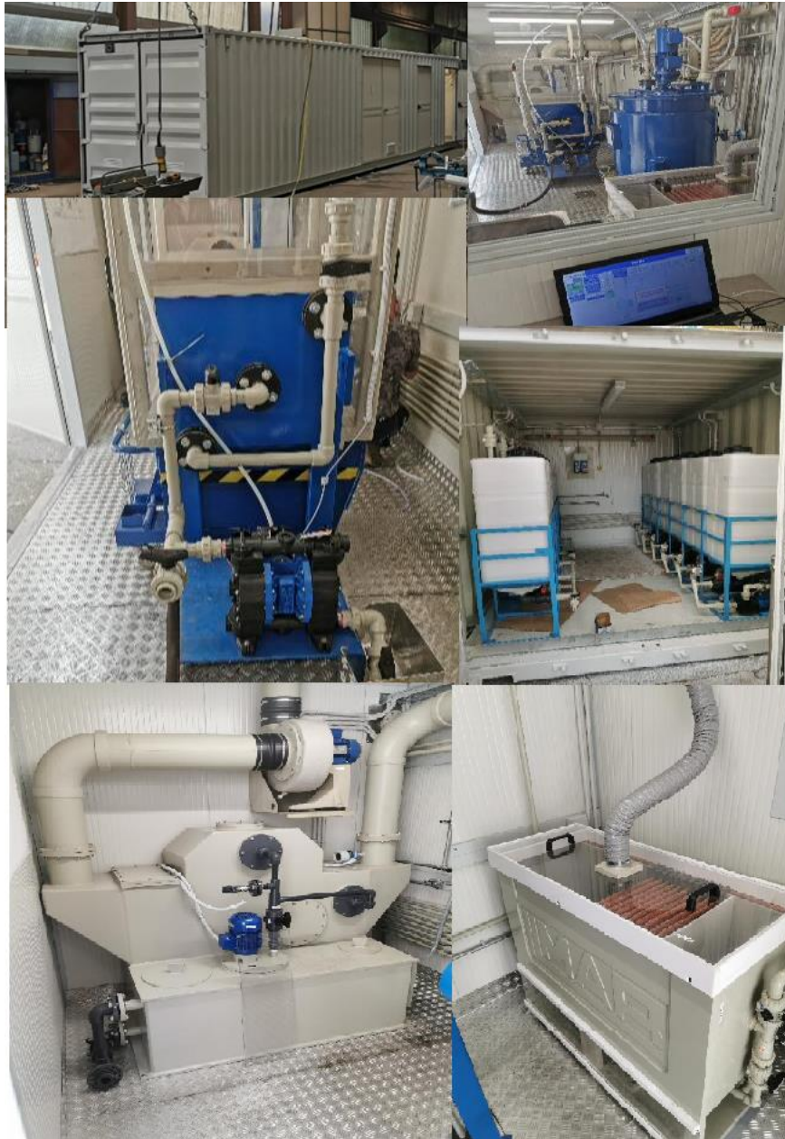
Figure 2: External and internal views of Fenix's hydrometallurgical plant
